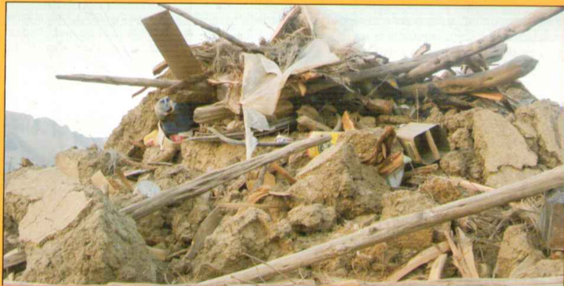
Figure : Aftermaths of earthquake in district Ziarat and Pishin
